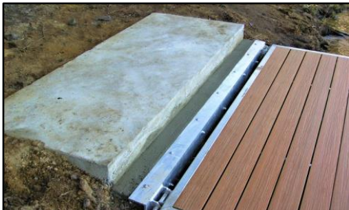
Concrete Angle on New Concrete
