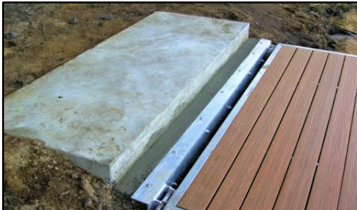
Concrete Angle on New Concrete
