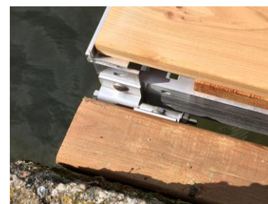
Ramp to Shore Hinge
